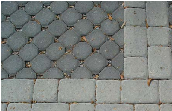
"Ecostone" Porous Paving with Conc. Cobble Surround
