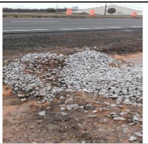
Figure 2 (Along Ox Road)
