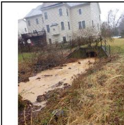
Figure 19 (Outfall at the back of Kelley Drive)
