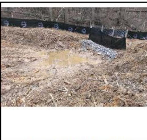
Figure 6 ( Near Tree Stockpile (Sheet U(2)))
