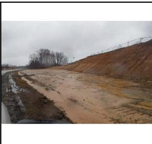
Figure 20 (Along Ox Road)
