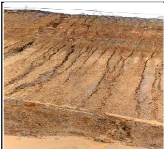
Figure 3 (Along Ox Road)
