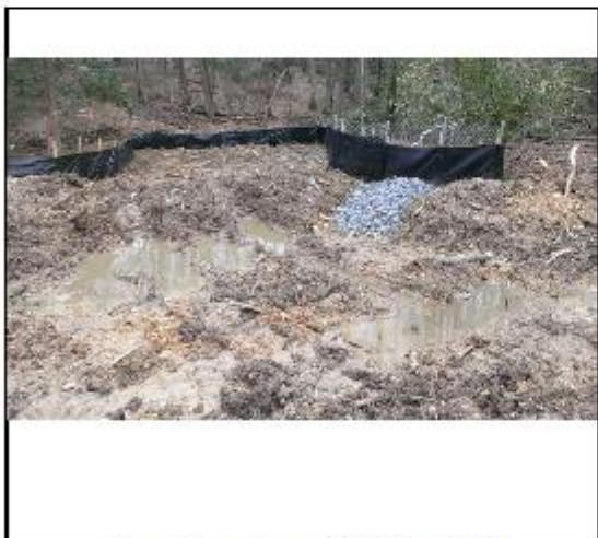
Figure 7 ( Near Tree Stockpile (Sheet U(2)))
