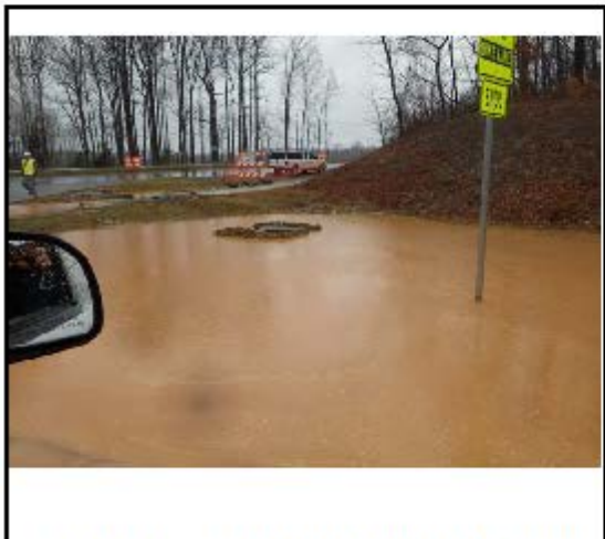
Figure 15 (Intersection of Mason Pond Drive and Ox Road)
