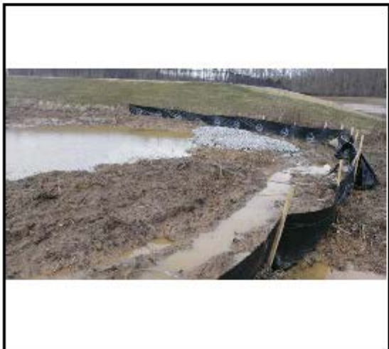
Figure 13 (Sediment Trap behind field 5)
