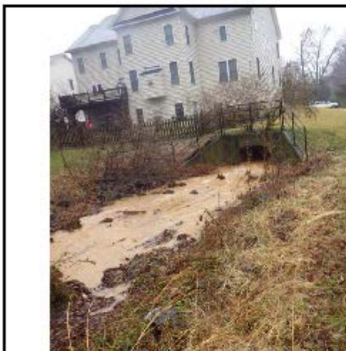
Figure 19 (Outfall at the back of Kelley Drive)
