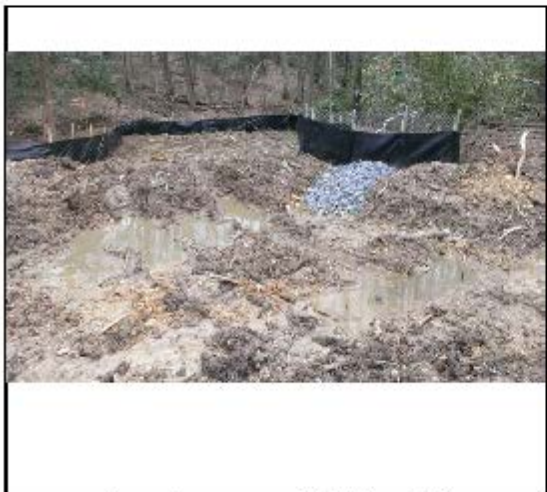
Figure 7 (Near Tree Stockpile (Sheet U(2)))
