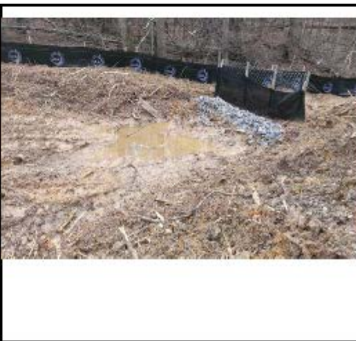
Figure 6 (Near Tree Stockpile (Sheet U(2)))
