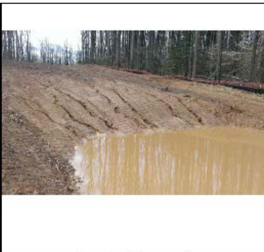
Figure 8 (Sediment Trap 3)
